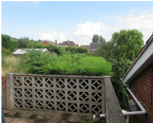
Photo taken facing east from elevated patio of No 6
